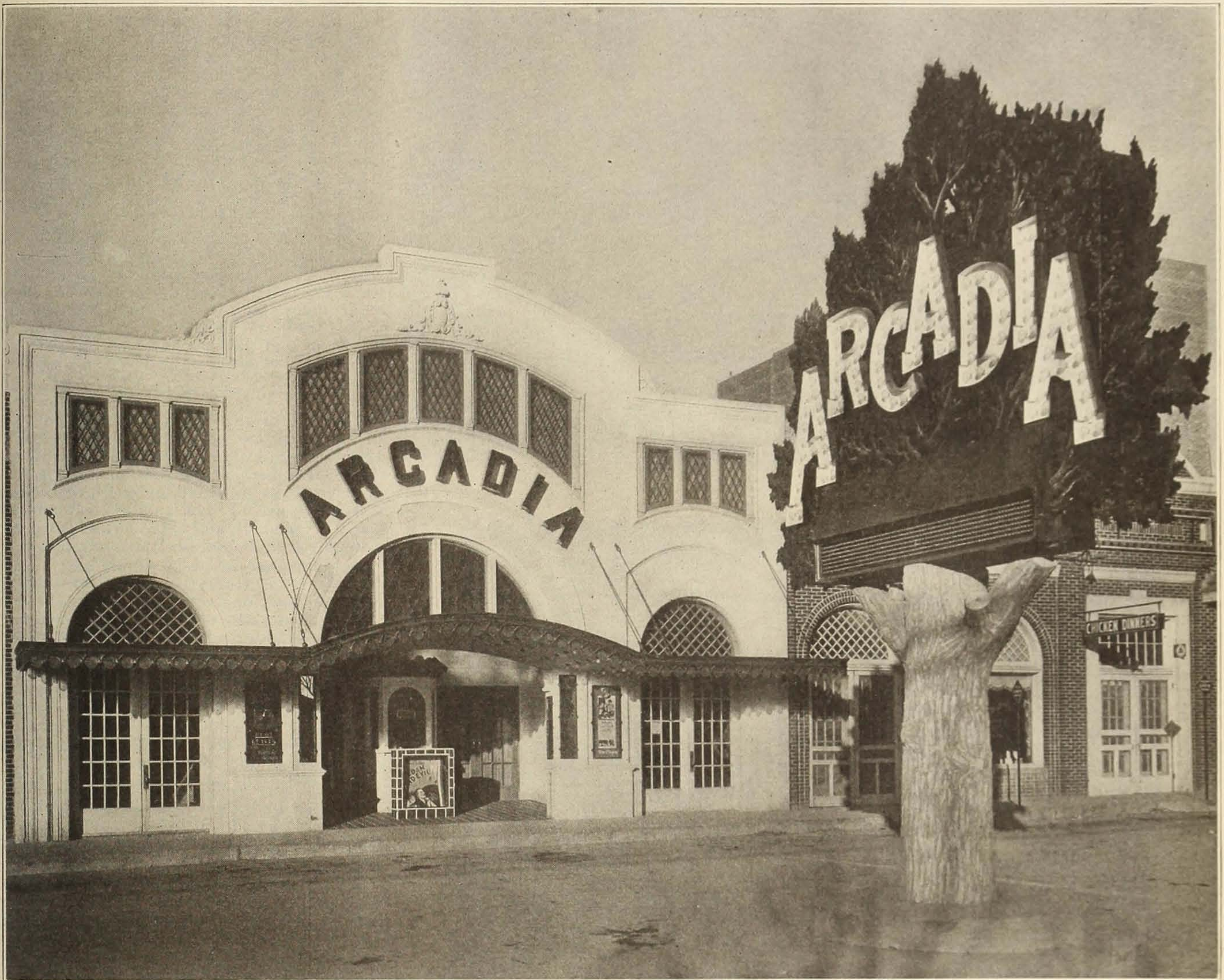
The entrance to the Arcadia. The tree stump is of concrete reinforced with railroad rails, while the branches are of angle iron bolted to the rails. Surely, no tree in Arcadia was ever stronger.
