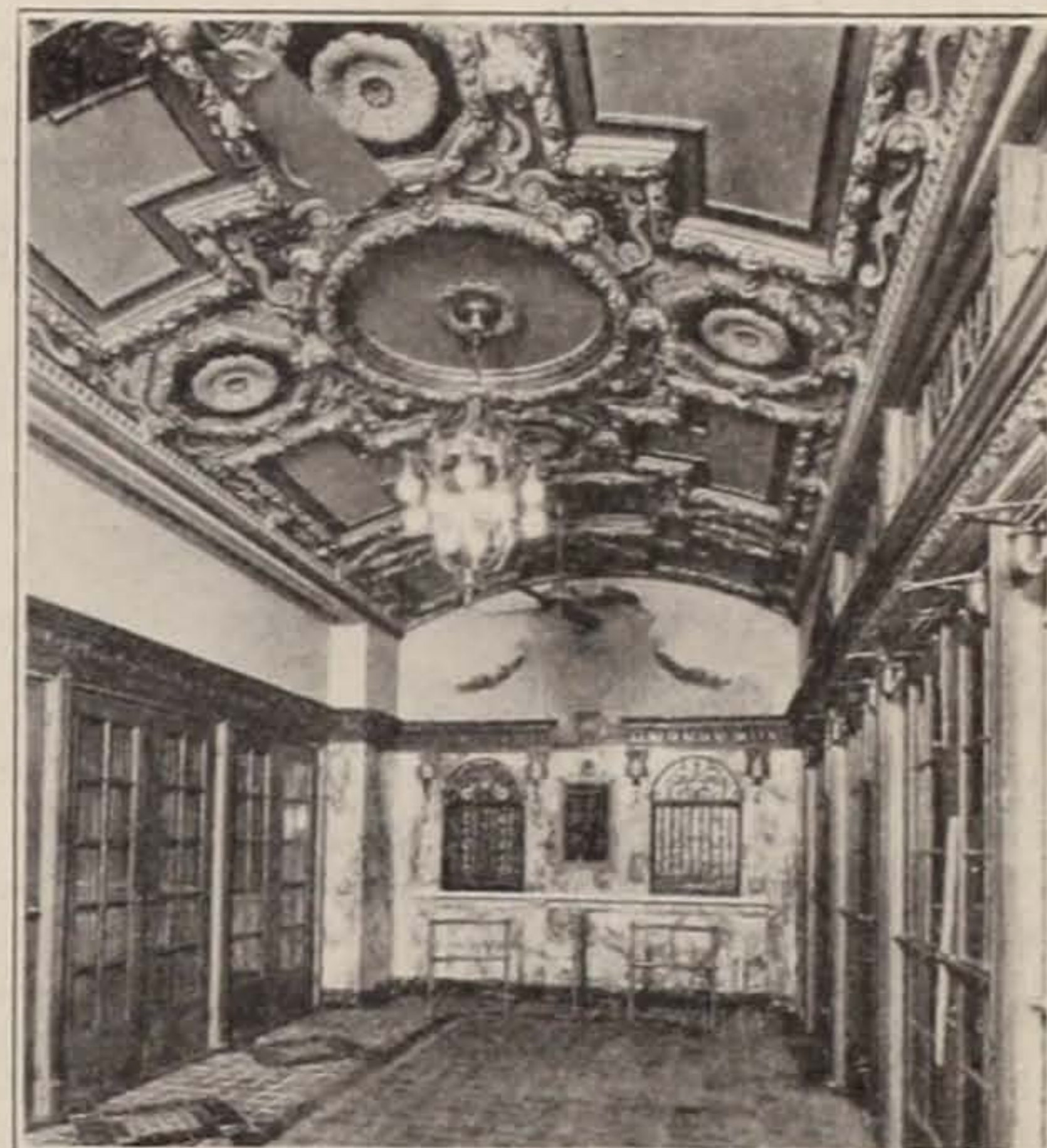
Entrance lobby of the Majestic, showing faience tile floor, violet marble wainscoting and richly ornamented coffer ceiling.
