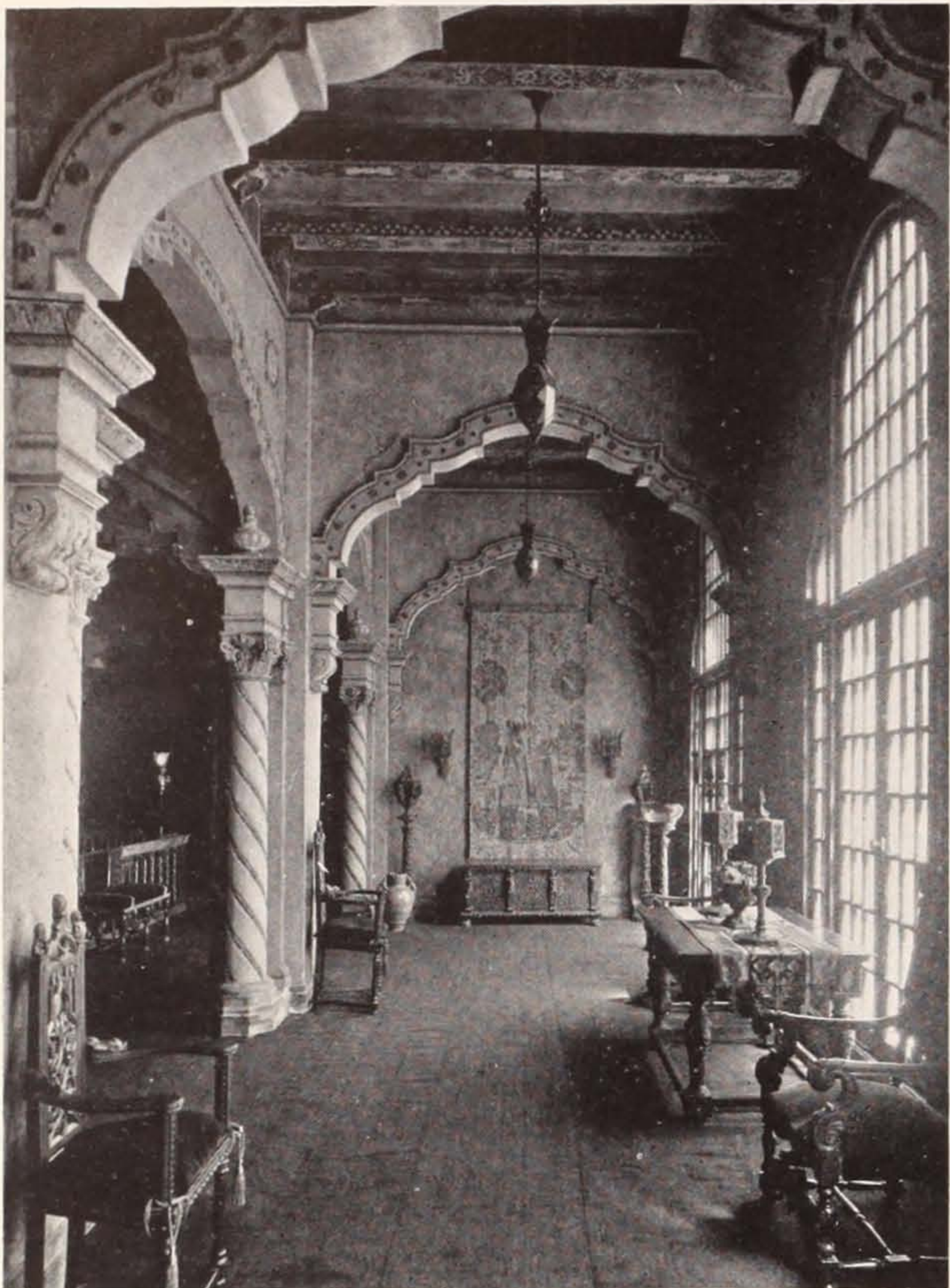
PORTION OF MEZZANINE OF THE OLYMPIA THEATRE, MIAMI, FLORIDA, SHOWING GENUINE AND REPLICAS OF ANTIQUES JOHN EBERSON, Architect
