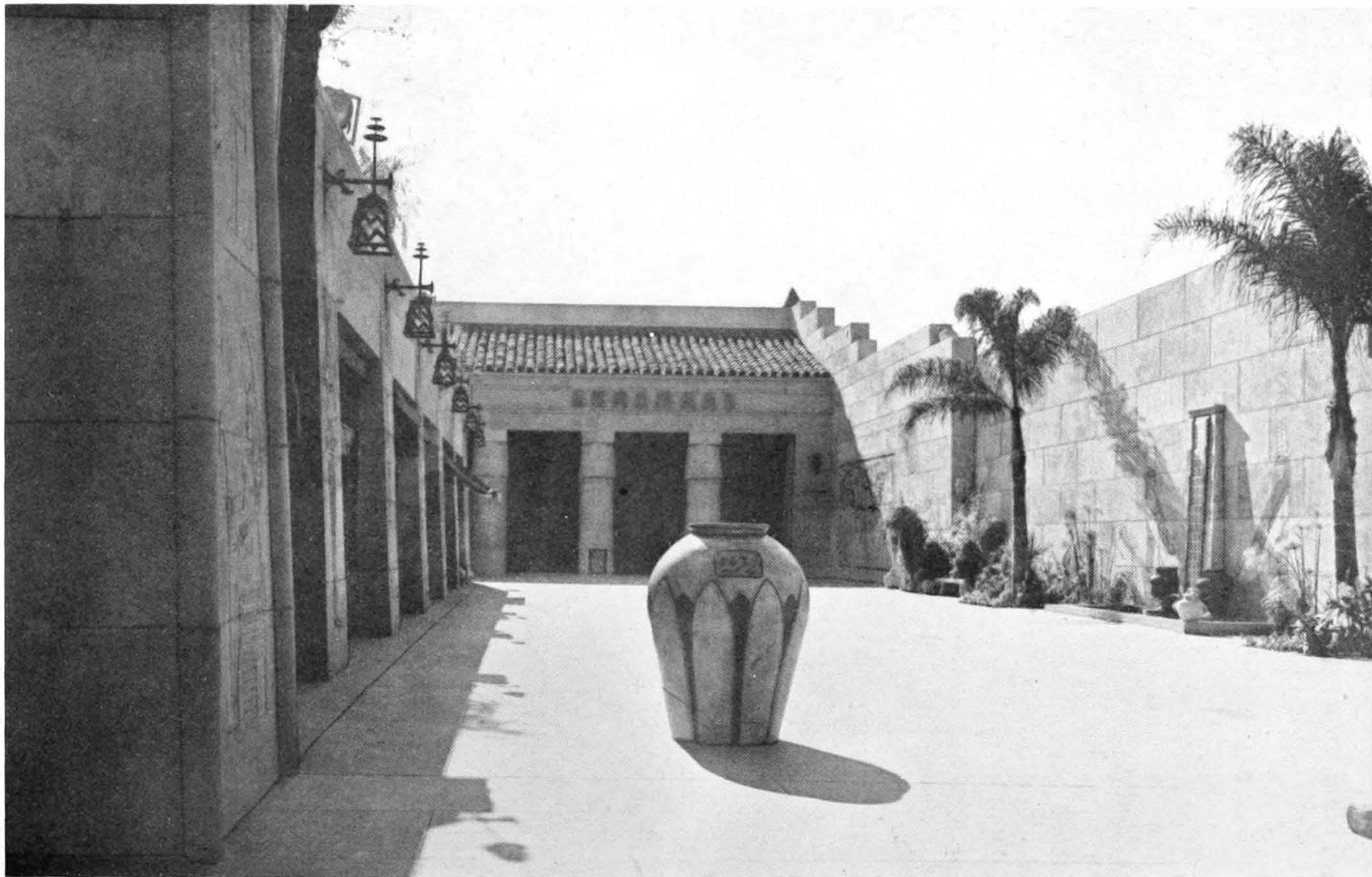
APPROACH TO THEATER, SHOWING FORECOURT AND SHOPS, GRAUMAN THEATER HOLLYWOOD MEYER & HOLLER, ARCHITECTS
