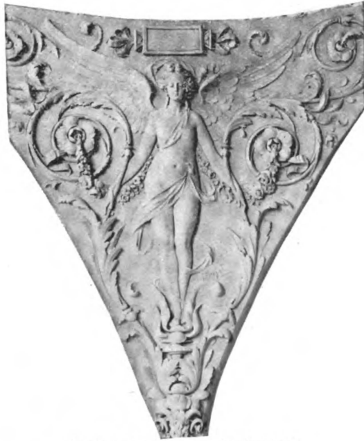
DETAIL OF PROSCENIUM ARCH,
