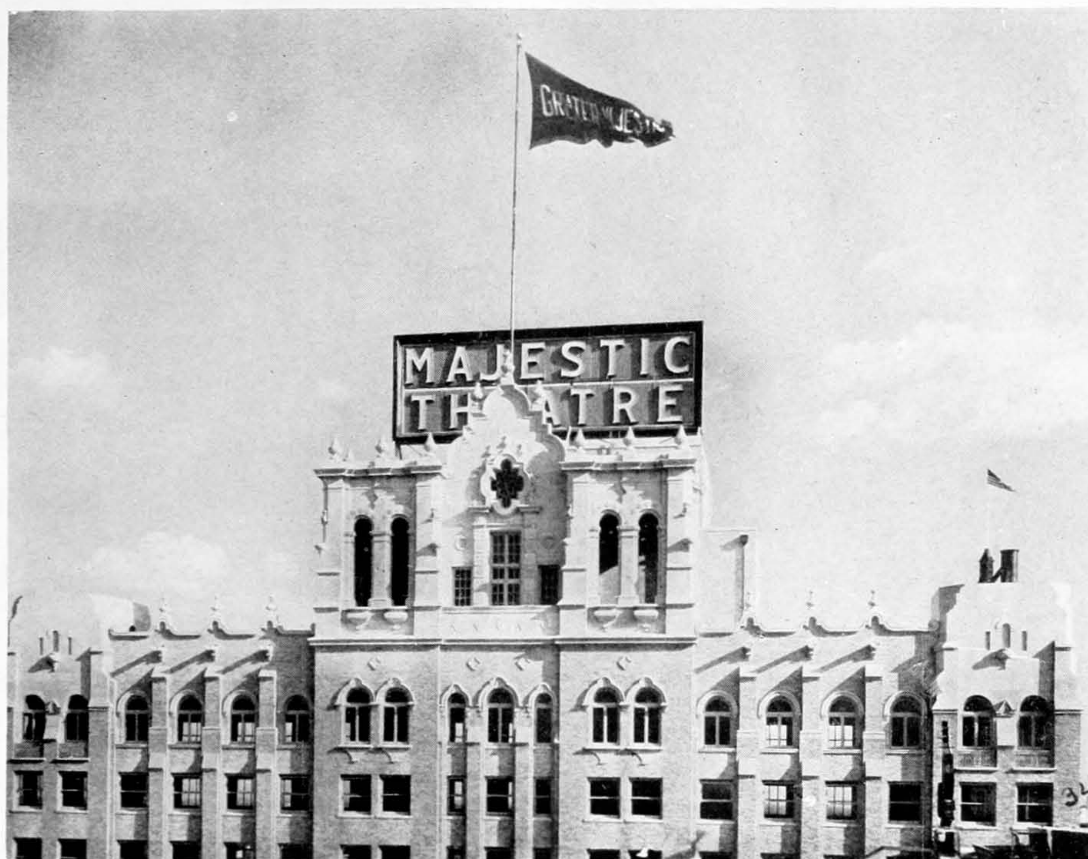
Top of the Greater Majestic office and theatre building, an 18-story structure in stone, showing Karl Hoblitzelle's pent house studio and sign which is visible for 50 miles.
