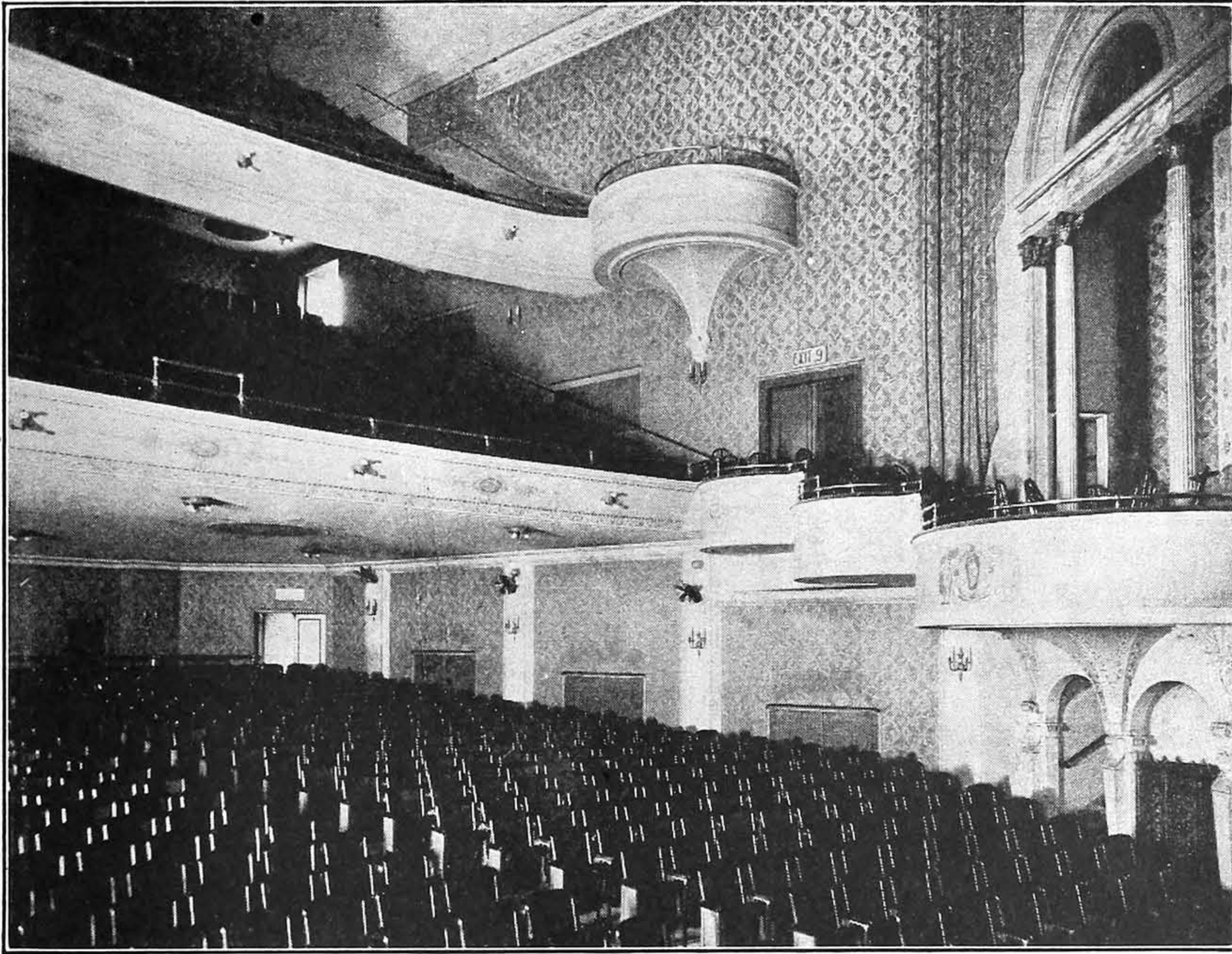
National Theatre, Washington, D. C., Warren & Wetmore, Architects—All side walls of this theatre were finished in Johns-Manville Acoustical Treatment. The installation, which was made after the theatre had been completed and occupied, shows the decorative possibilities of the acoustical material, and that it may be applied without mutilation of architectural details.
