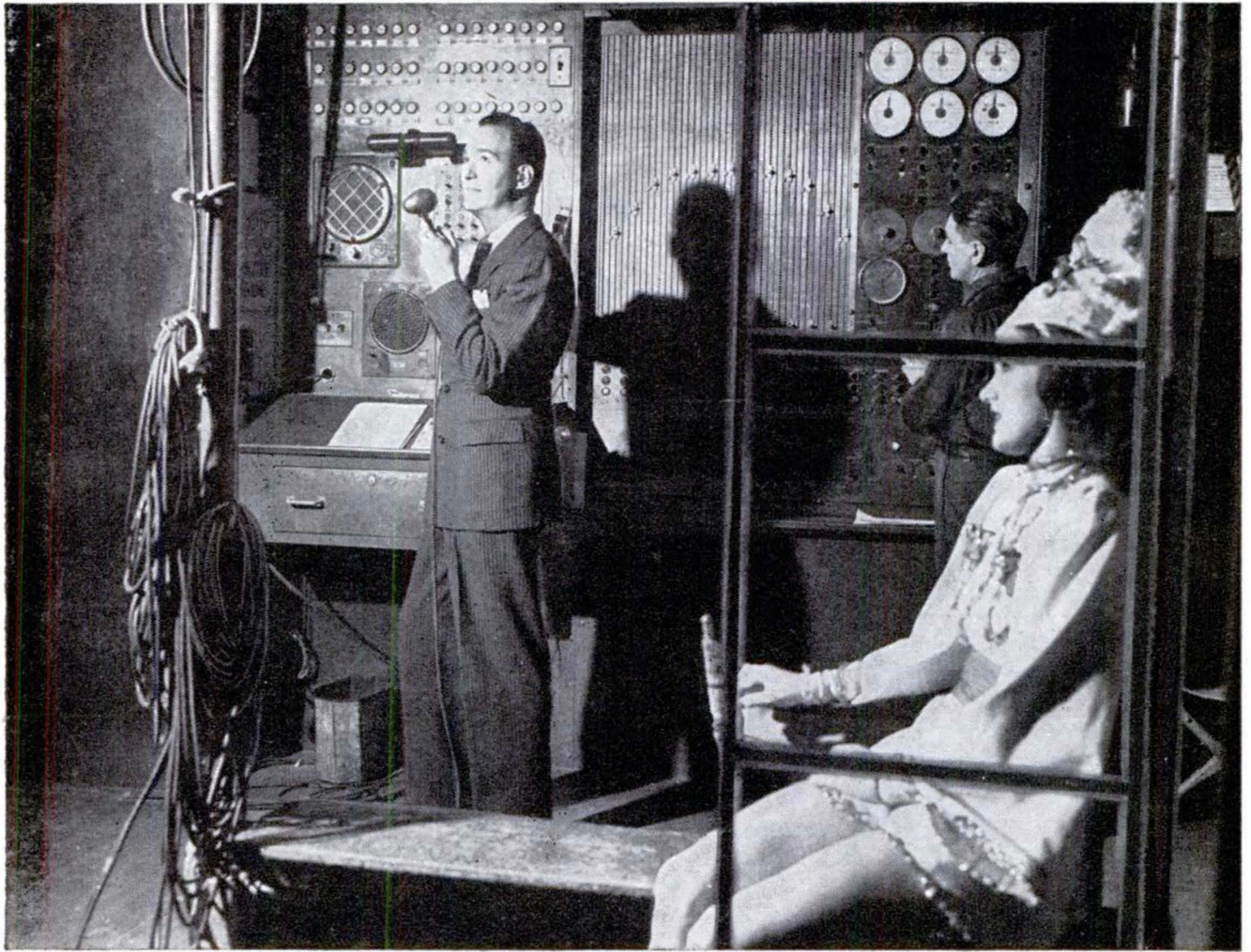
Central panel on stage-manager's control board regulates giant curtain; sliding buttons show preset pattern
