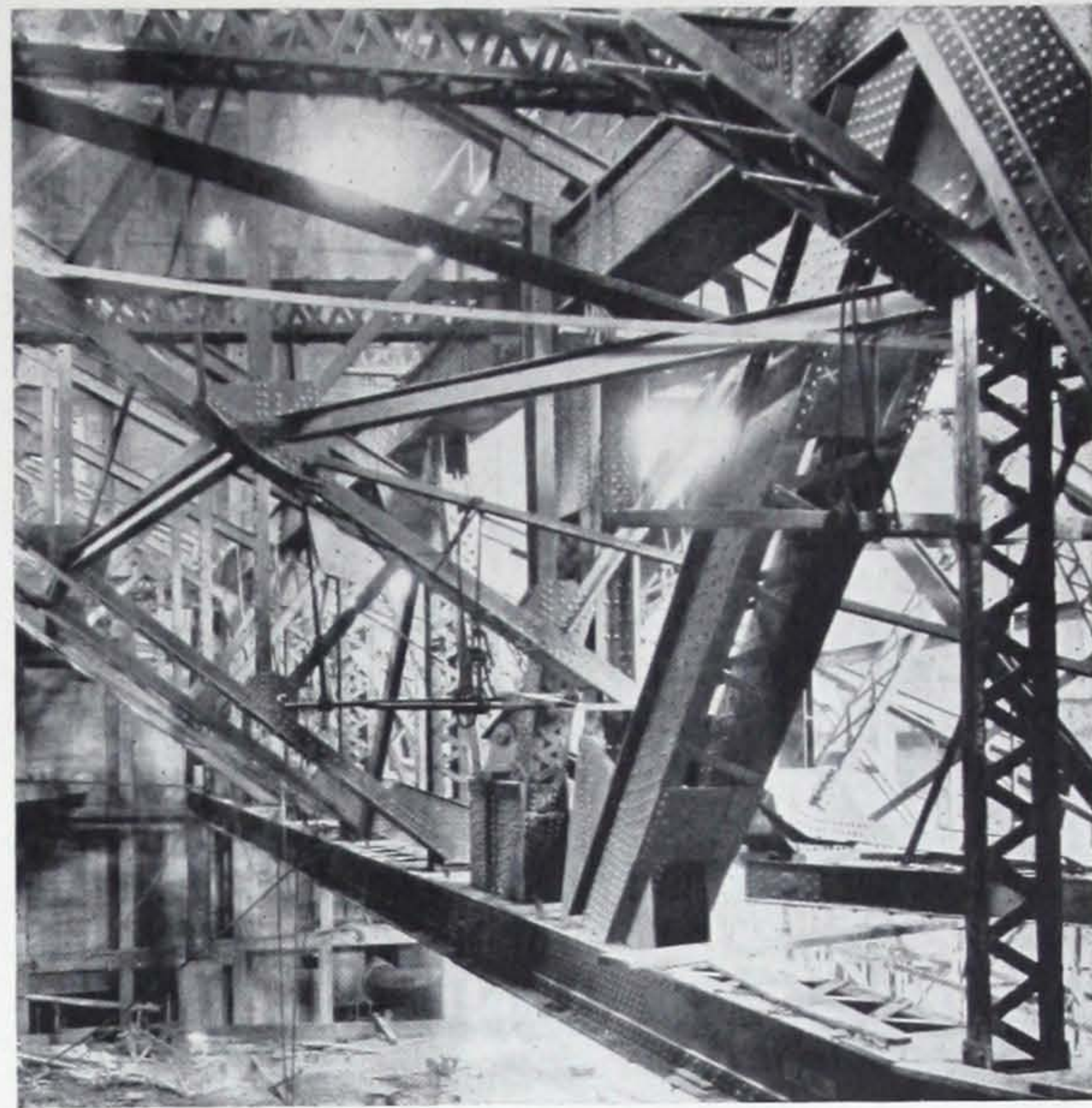
MAIN BALCONY TRUSS SHOWING INTRICACY OF CONNECTION DETAILS AND PIN CONNECTION OF JACK TRUSS TO STEEL CASTING ON MAIN TRUSS. ELECTRIC WELDING WAS USED TO OBTAIN METAL-TO-METAL CONTACT WHERE INCLINED SURFACES MADE IT DIFFICULT TO MILL ACCURATELY
