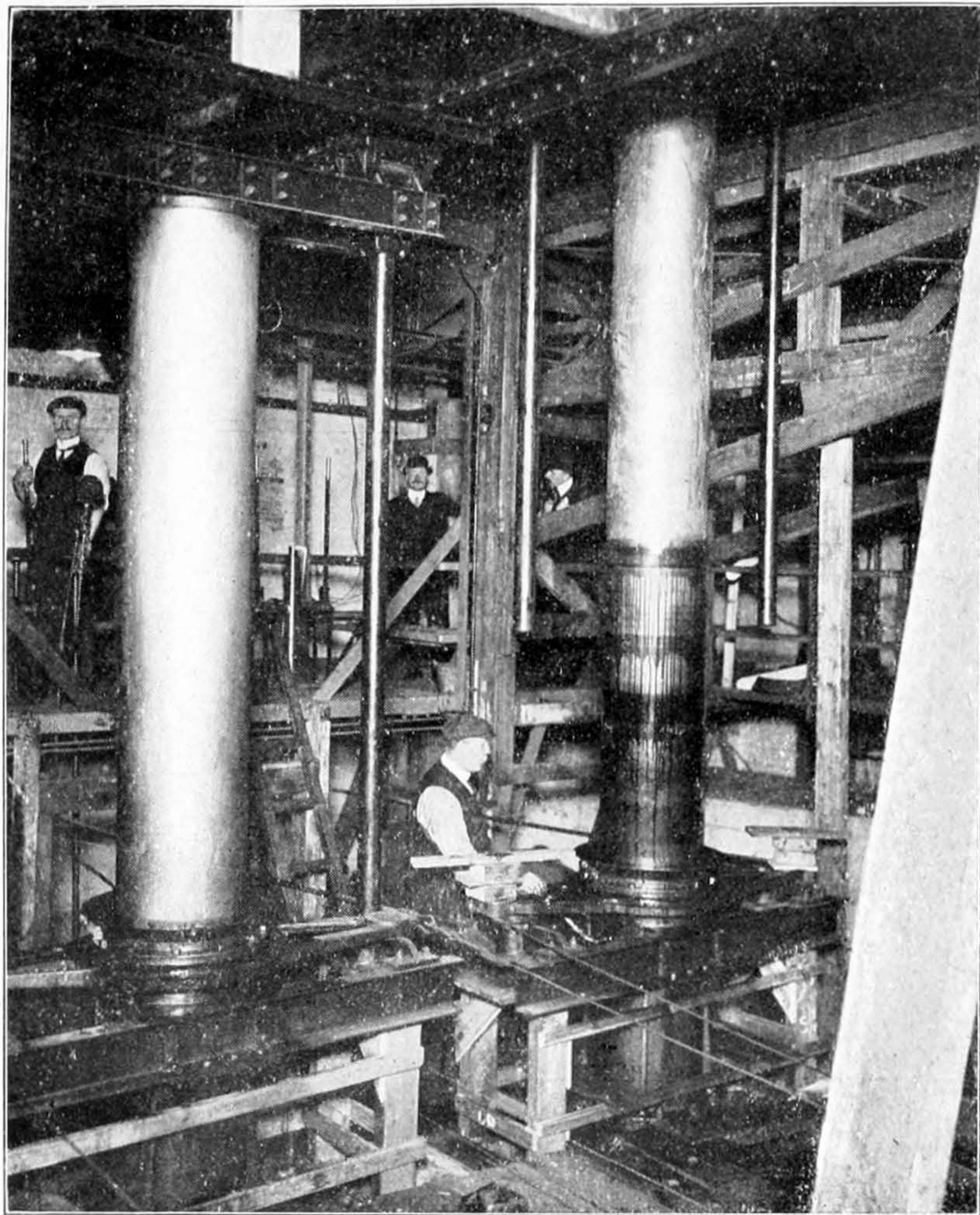
THE UNDERSIDE OF THE STAGE, Showing the massive plungers.
