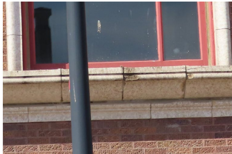
SPALLED UNITS
