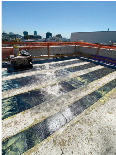
Fig. 3. Early coordination between Structural Focus and various FRP suppliers was required to ensure the diaphragm FRP strengthening design requirements specified on the structural drawings were feasible.
