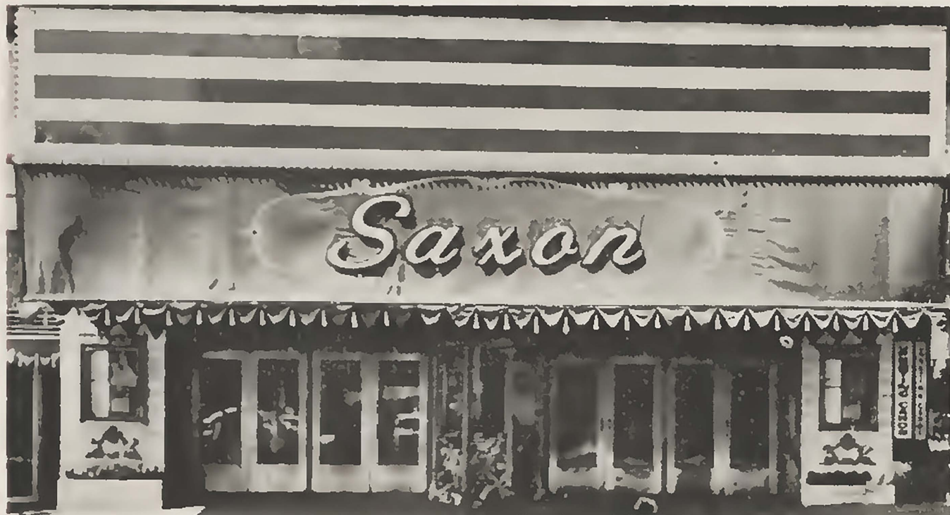
A new marquee was erected over the entrance of the former Midland Theatre, now the Saxon, in Kansas City, Mo., and a canopy bearing the theatre name suspended beneath it. The color scheme is green and gold. The boxoffice remains in the center, but rough stone planters were added on either side.
